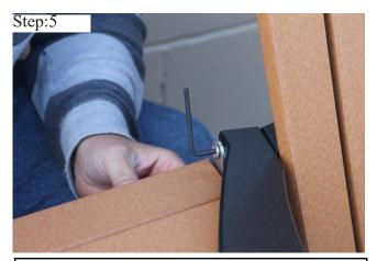
Install bolt provided in kit assembly bag. Connect the bracket through the arm and into the chair back. Repeat on the other chair.
