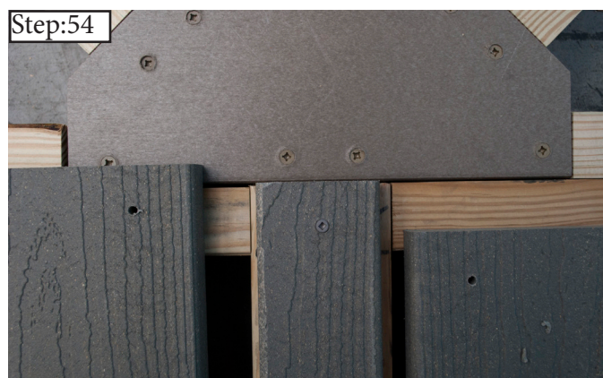
Step:54 Place the smaller Deck Board directly in the center as shown.
