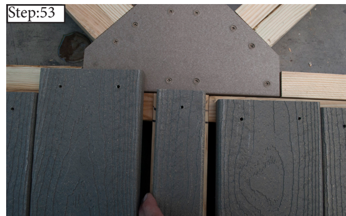
Step:53 Locate the smaller Deck Board and place in the center of the Floor Section.
