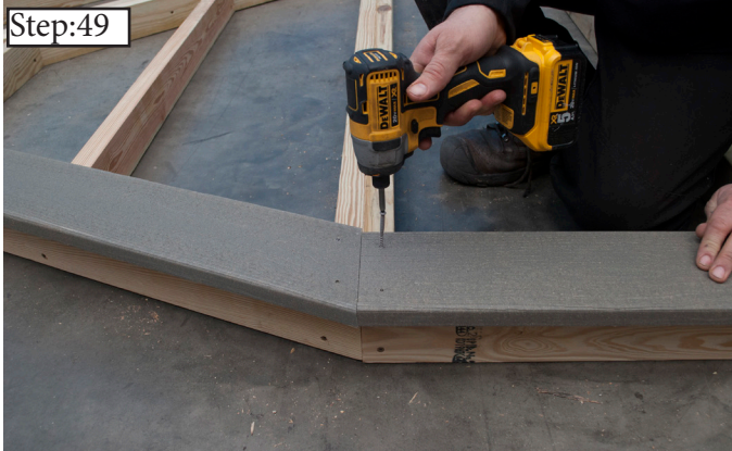
Step:49 Continue around the outside of the floor and place the adjacent Deck Board against the first Deck Board and fasten, as shown in Steps 46-48.
