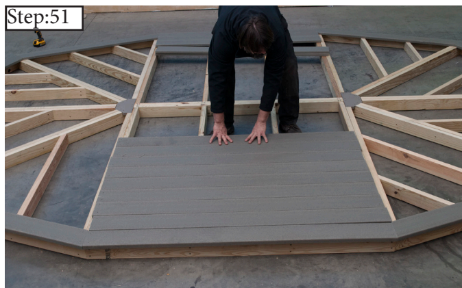
Step:51 Locate the rest of the Straight Cut Floor Deck Boards and place in line as shown.
