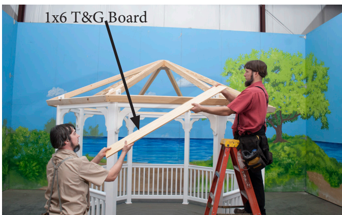
Locate the Tongue & Groove Boards, start with the longest one.
