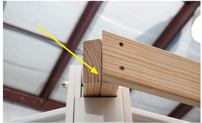
Place edge of Roof Band Board in center of the Rafter.
