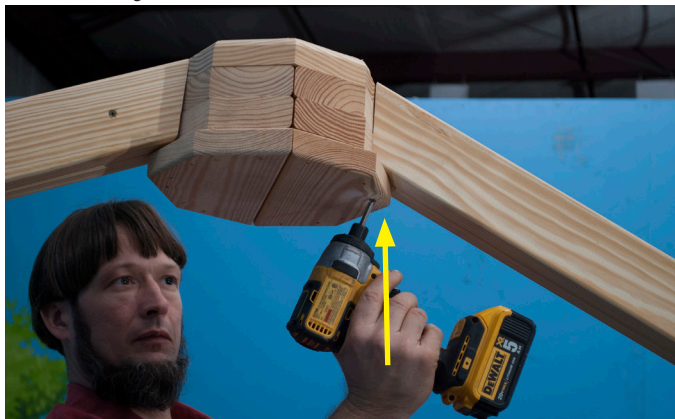
Attach Rafters to Compression Ring from the bottom up using two (2) 3" Screws per Rafter.
