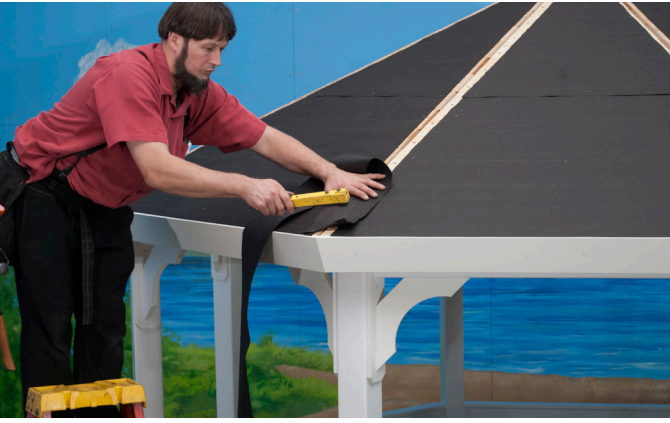
Center the Ridge Tar Paper and fasten at the bottom using a Hammer Tacker.
