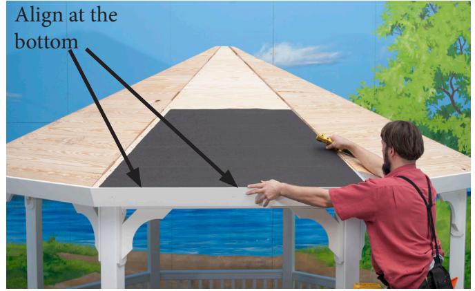
Start by placing the Large piece at the bottom as shown.
