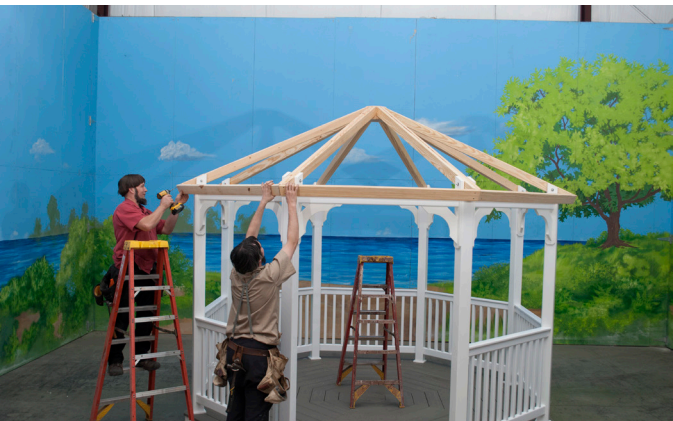
Continue by attaching all remaining Roof Band Boards to Rafters.
