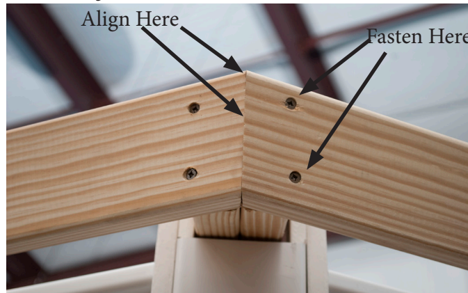
Align the end with the previously installed Roof Band Board and attach with two (2) 3" screws.
