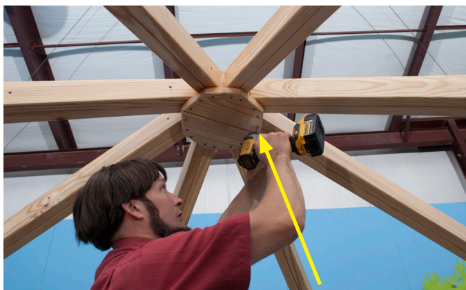
Ensure all Rafters are fastened to the Compression Ring. Two (2) 3" Screws into each Rafter.
