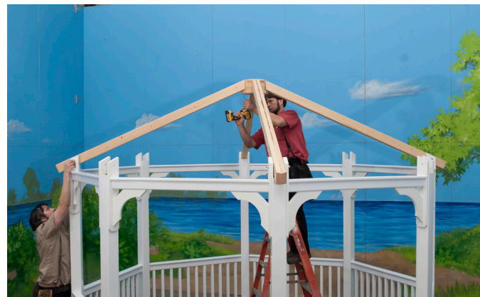
Continue to install the next Rafter opposite the third Rafter.
