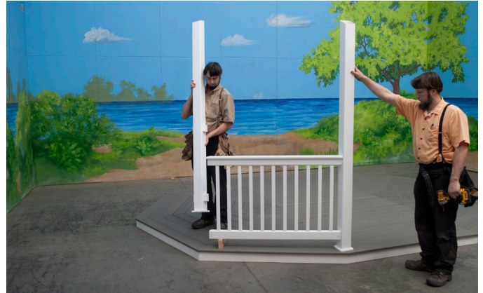
Locate a Standard Post with Four Railing Inserts
