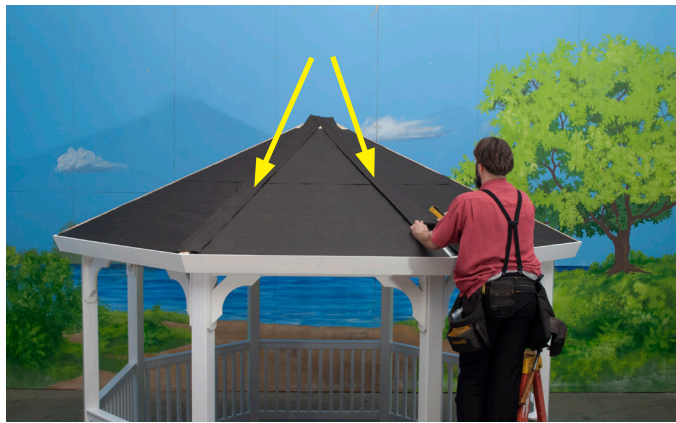
Install remaining Ridge Tar Paper, as shown in previous steps.
