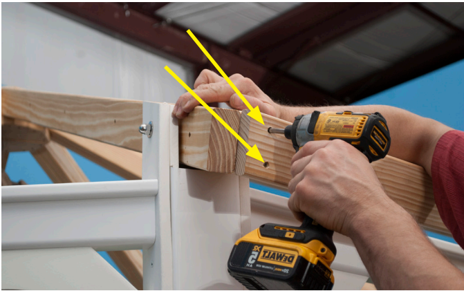
Fasten the Roof Band Board to the Rafter using two (2) 3" Screws through pre-drilled holes.
