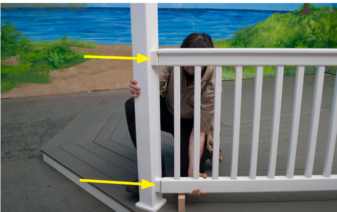
Slide top and bottom Railing pieces onto Railing Inserts as Shown.
