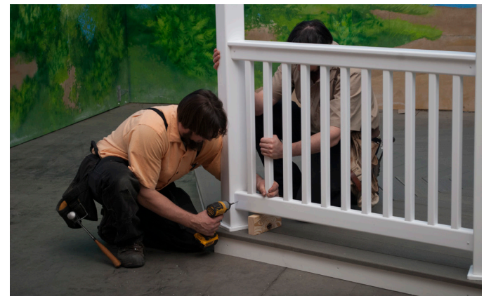
Push Railing sections tight against post and attach using one (1) 1" Pan Head Screw through pre-drilled hole, as shown.
