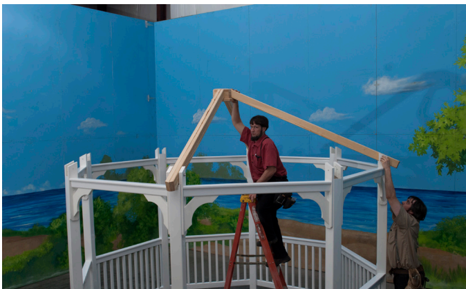
Install another Rafter as Shown in previous steps.
