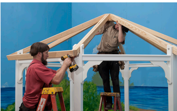
Push up on the Double Rafters in the center until the Roof Band Board is center of the Rafter and fasten using two (2) 3" Screws through pre-drilled holes.
