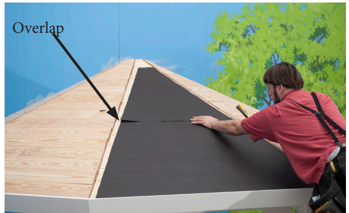
Place the Small piece of Tar Paper on top of the Large piece and overlap the Tar Paper by 2 inches. Fasten Tar Paper, as shown in previous steps.
