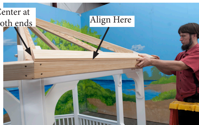
Center Tongue & Groove Board at Rafter Splice, align flush with Band Board.
