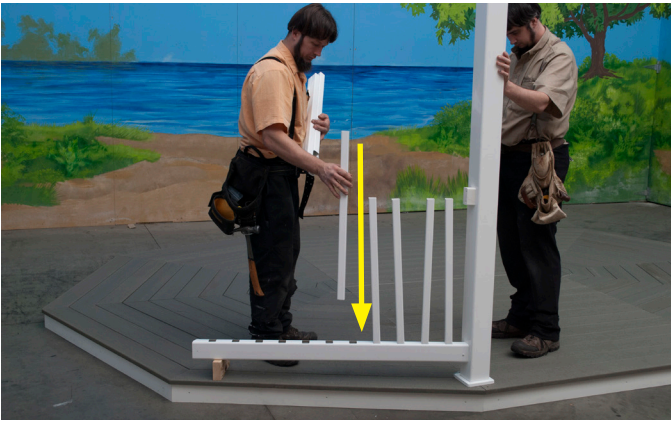
Place the Spindles into the Bottom Rail.
