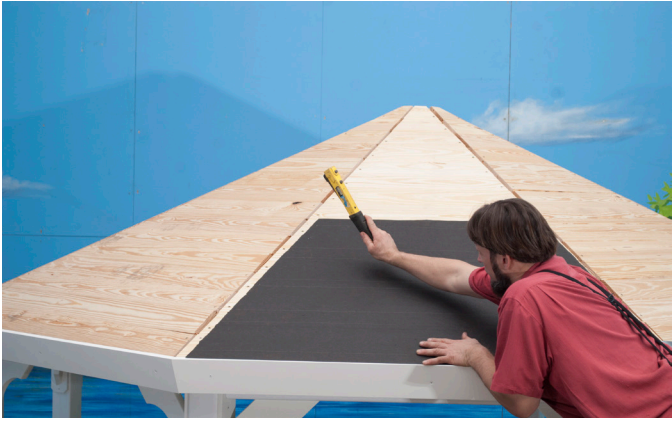
Fasten Tar Paper to Tongue & Groove Boards using a Hammer Tacker.
