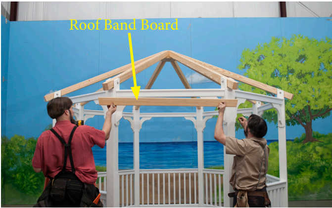
Locate the Roof Band Board.
