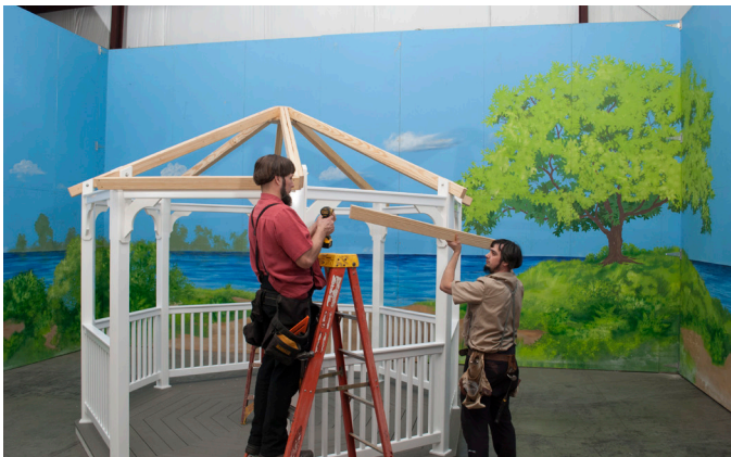
Lift next Roof Band Board into place.
