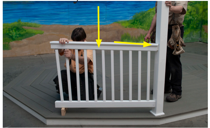
Working your way across place the Spindles into the holes of the T Rail.
