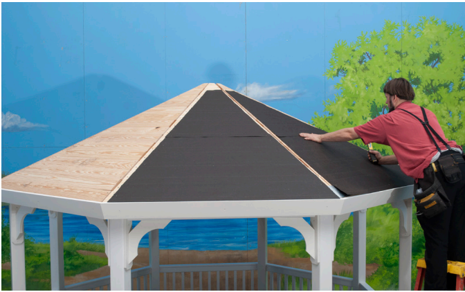
Install all remaining Tar Paper on roof.
