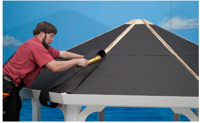
Roll Tar Paper up the Ridge and fasten Tar Paper to Ridge approximately every 6 inches.
