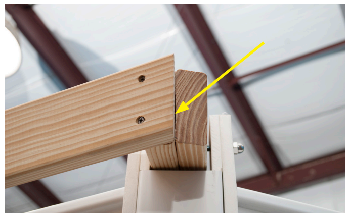
Roof Band Board aligned and attached.
