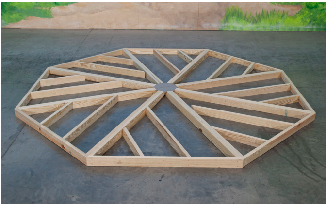
Place remaining Diagonal Floor Joists in Place as shown.
