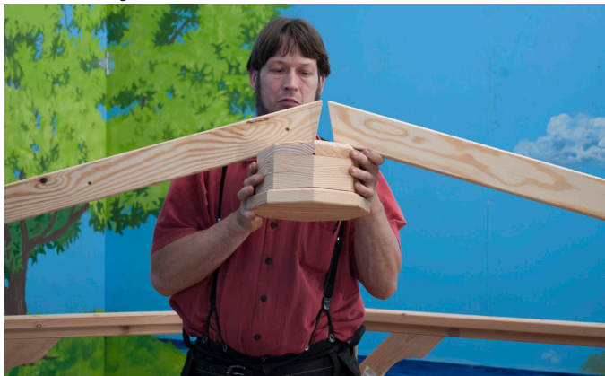
Locate the Compression Ring. Lift Compression Ring into place.
