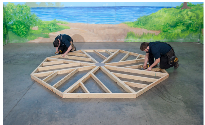
Fasten remaining Diagonal Floor Joist using previous steps.
