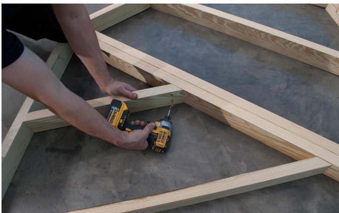
Fasten the 45° angled end to the Double 2x4 Joist using two (2) 3" Screws through pre-drilled holes, as shown.
