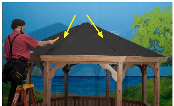
Install remaining Ridge Tar Paper, as shown in previous steps.
