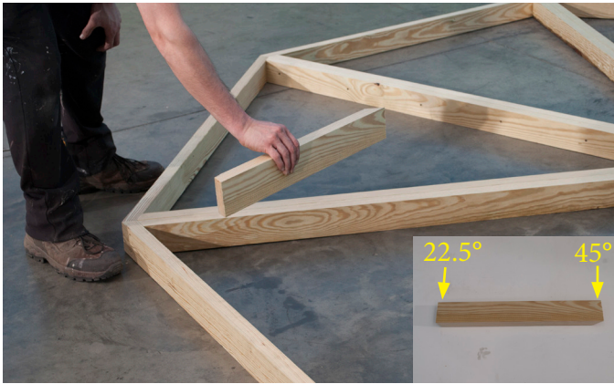
Locate the Diagonal Floor Joists.
