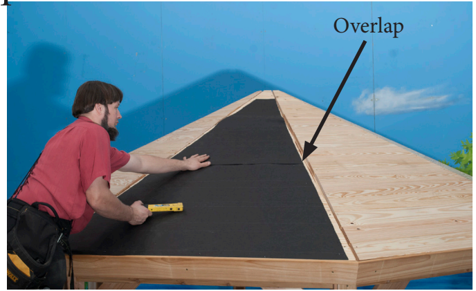
Place the Small Tar Paper piece on the top side. Overlap the Small piece over the Large piece by 2". Fasten using a Hammer Tacker.
