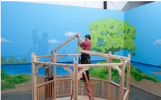
Install the Rafter directly opposite of the previously installed Rafter, as shown in previous steps.
