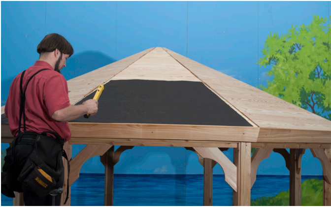
Fasten Tar Paper to T & G using a Hammer Tacker.
