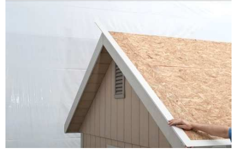
(187) Overlap the gable piece over the bottom piece and nail only the bottom.
