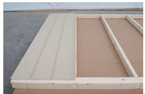
(49) Ensure that stud is parallel with siding, before nailing. Then firmly attach siding section along all edges and into each wall stud, using an 8" to 12" nail spacing.
