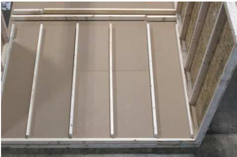
(89) Locate and lay out the parts to assemble the gable wall.
