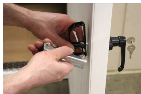
(174) Attach D-handle as shown using a 5/32 Allan Wrench. Adjust as needed.
