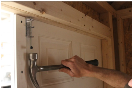
(170) Pull the left door in, tight against the frame, then make a mark for the inside latch pin. Repeat on the bottom.
