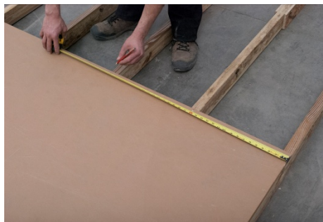
(32) Before you finish attaching the first row flooring to the joist, make marks 12" on center for a guide to adjust the joist when nailing. Then finish nailing the first row flooring.
