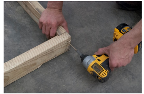
(18) Attach the band board, using 3" screws, through the pre-drilled holes. Make sure the floor joists are flush with the band board as shown in next step.
