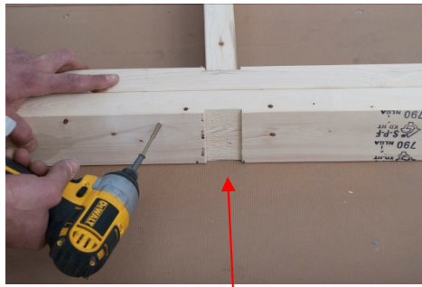
(42) Before fastening the double top wall plate, ensure that dado grooves align with wall studs, and are faced outward.
