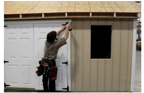
(169) Finish fastening the rest of the hinges, using previous steps.
