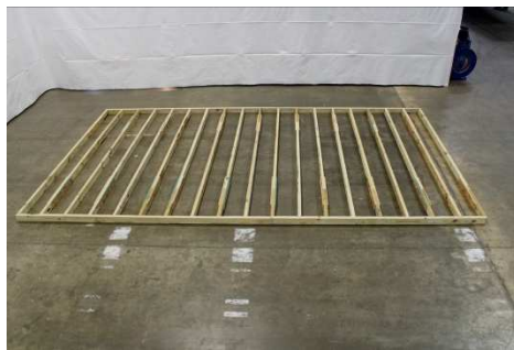
(23) Continue until floor is complete.
