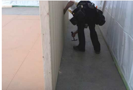
(72) Repeat along the rest of the wall.
