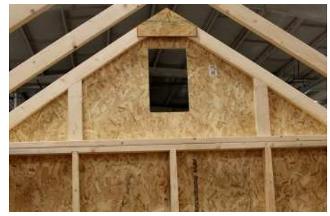
(130) Fasten the other gable brace on this gable, then repeat for opposite gable. Next, fasten the siding splices to the gable braces on the outside.
