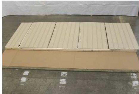
(54) Repeat previous steps for the rest of the siding.
