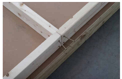
(40) Repeat the process for the rest of the bottom plate; but use four 3" screws as shown, for any splice.
