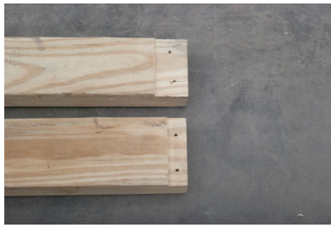
(17) The band boards have dado grooves precut to ensure proper joist placement. The narrow grooves should both be placed at the splice, and the wider grooves at the ends.
