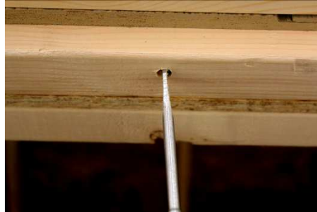
(171) Drill a hole, with 5/16" drill bit, using the pre-made marks.
