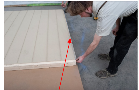
(55) Snap a line, even with the edge of the wall frame, then move to next step.
