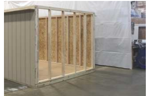
(91) Set the gable wall.
