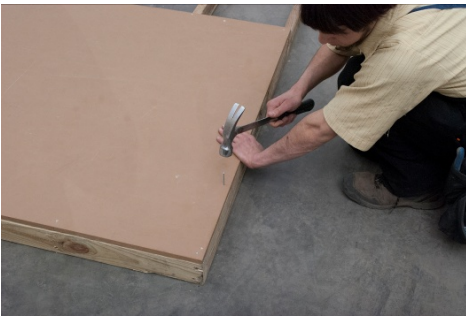
(28) Nail along the gable, making sure flooring is flush with the floor joist. Use an 8" to 12" nail spacing.
