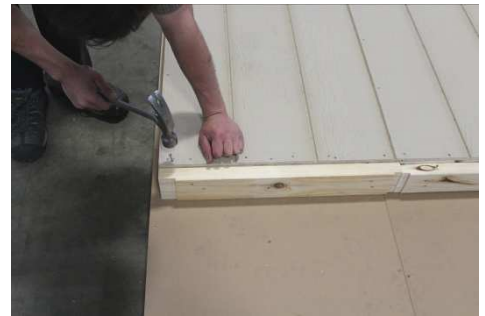
(46) Nail this corner with one 2" nail, before moving to the next step.
