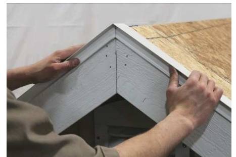
(190) Bend around the top as shown. This top piece should overlap the bottom piece. Do not fasten it till the bottom piece is installed on the other side. Finish installing the rest of the drip edge.
