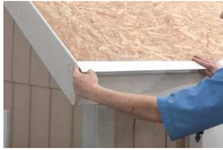
(186) Keep drip edge flush with the gable as shown, then nail every 12 to 14 inches, using roofing nails. (Nails not included.) Repeat for the next pieces, overlapping about one inch, and keeping the last piece flush with the other gable.
