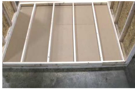
(90) Attach all wall studs to top and bottom and wall plates.
