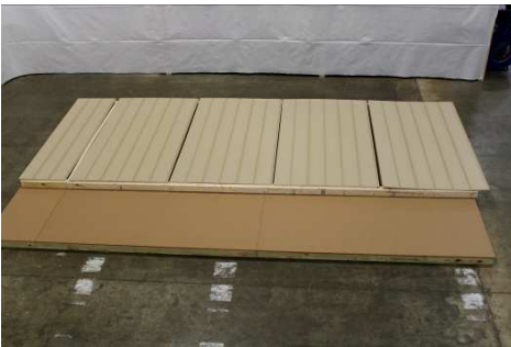
(44) Lay out siding as shown here, with the overlap towards the left. (Refer to drawings)
