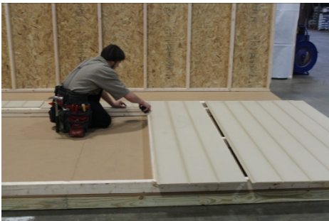
(83) Repeat for the other door piece. (Siding spacing from left to right to be spaced at 72")
