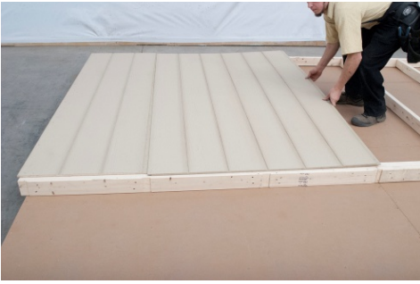
(50) Put the next piece in place, flush with the previous piece.
