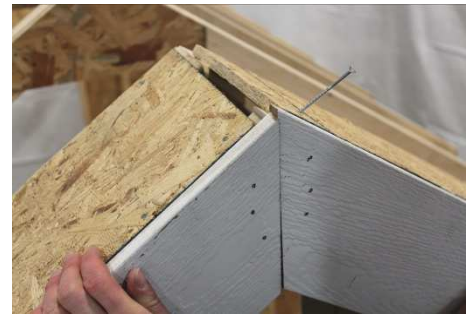
(124) Incorrect! Before fastening the overhangs on the top, make sure the splice is uniform, as shown in next step.
