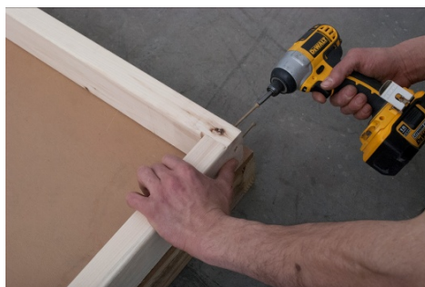
(39) Insert two 3" screws through the pre-drilled holes to attach bottom plate to each wall stud. Make sure bottom plate and wall studs are flush.
