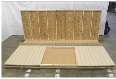
(87) Cut the end of the siding, repeating steps (55 to 57) Then, install soffit, repeating steps (59 to 64) NOTE: Install soffit, starting on the same end as the previous wall.
