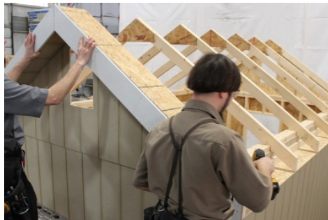
(123) Install right gable overhang, repeating previous steps.
