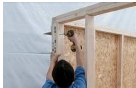
(93) Align gable wall framing flush with back wall framing and attach using 3" screws, every 12 to 14 inches. Repeat the process on front side.
