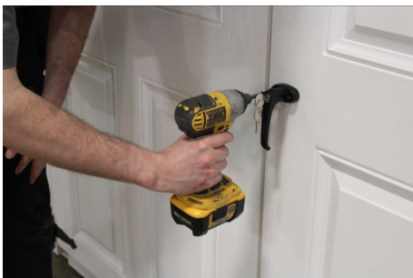
(173) Install latch using 2" black screws.
