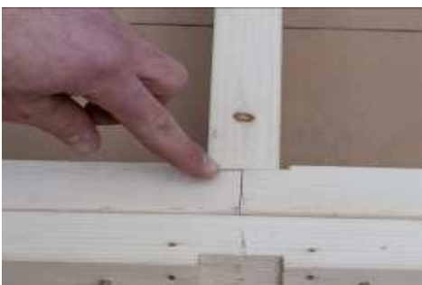
(38) Be sure to alternate the double, top wall plate splices.
