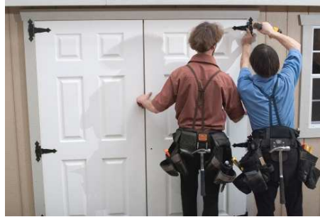
(168) Repeat for the right door, again; making sure you keep the top of the door down from the trim, approximately 1/4".
